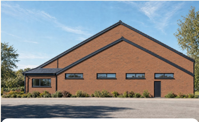
NORTH SIDE North elevation and approach.
