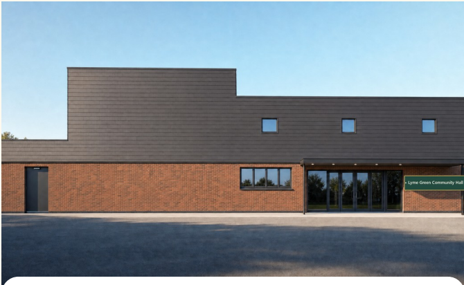
EAST ENTRANCE Main entrance with the plan-indicated canopy and hall sign.
